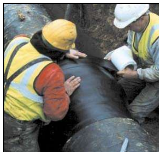
being overwrapped with Densoclad Tape...
