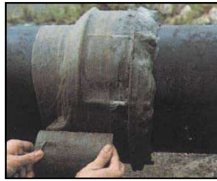
Overwrapping with Denso Tape
