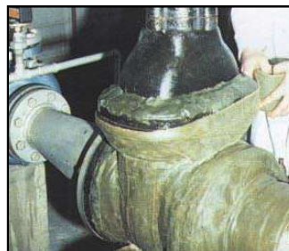
Overwrapping with Denso Tape
