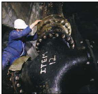
being overwrapped with Denso Tape...
