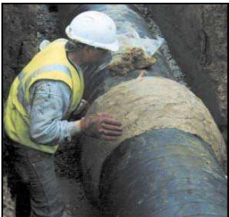
P2* application: Profiling Mastic on flange...
