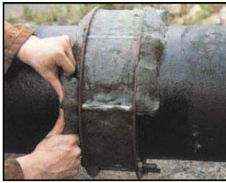
Profiling and infilling with Densyl Mastic.
