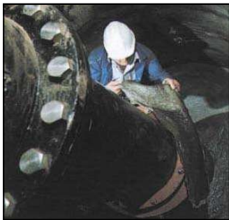
P1* application: Mastic Blanket on flange...
