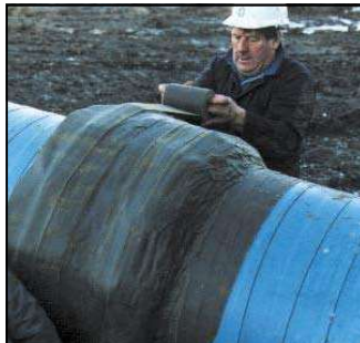
being overwrapped with Denso Tape...
