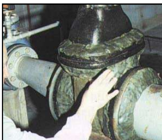
Profiling with Densyl Mastic.
