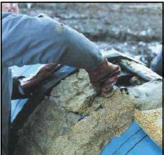
P1* application: Profiling Mastic on Tybar...
