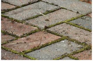
**Existing Installations**: Paving should be cleaned by water blasting, grit blasting or steam cleaning. The surface should then be allowed to dry before re-sanding and compacting the joints. It is preferable that, before sealing, the jointing sand is also dry. Do not apply when rain is expected. Typical Results Grey powder 2000 kg/m³ @ 25 °C < 2 minutes @ 25 °C 28 days Diesel, petrol and oil
