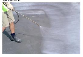
The clear or opaque film produced by TYL®-ChemCure Agent will degrade in direct sunlight within 21 days.
