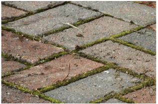
**Existing Installations**: Paving should be cleaned by water blasting, grit blasting or steam cleaning. The surface should then be allowed to dry before re-sanding and compacting the joints. It is preferable that, before sealing, the jointing sand is also dry. Do not apply when rain is expected.
